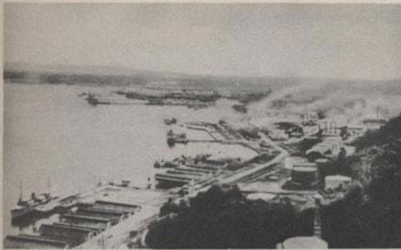
Docks and oil refineries, Balikpapan, Borneo.
